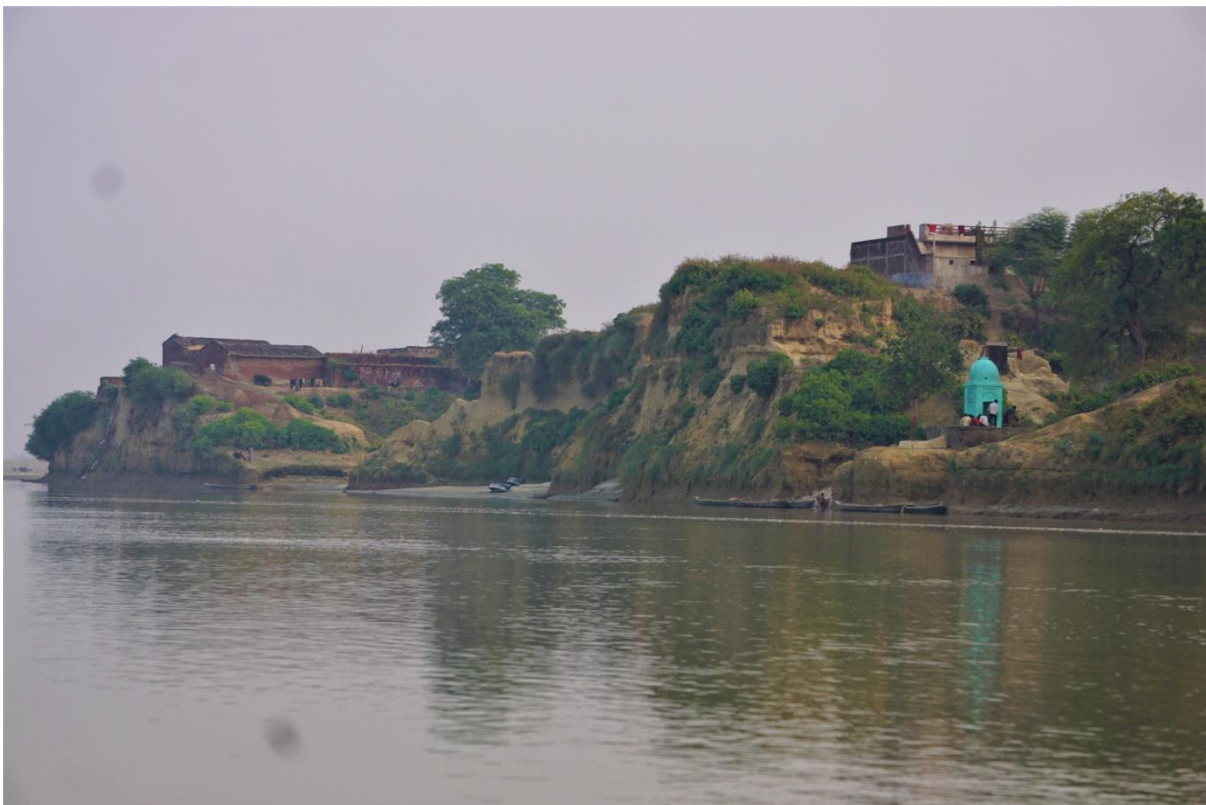
Image 55 : Erosion Prone Bank At Ujhni Khalsa Village
