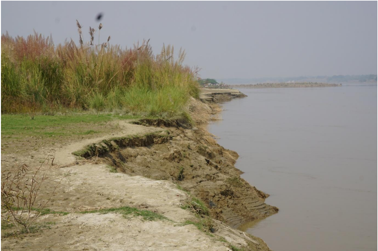
Image 56 : Eroded Site Near Afzalpur Saton And Kanthua Village
